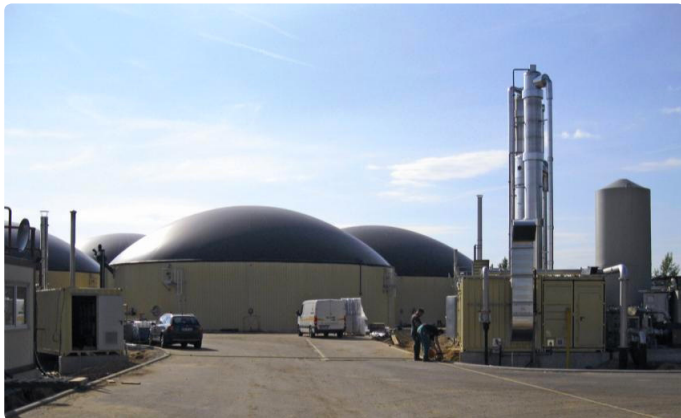
Biogas Plant Schöpstal
